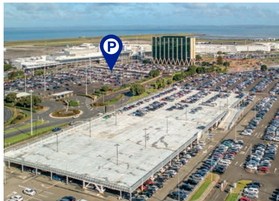
A new six-storey car park is planned for the International Terminal, featuring more than 3,000 car parks.
