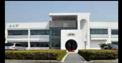
Changshu Manufacturing Facility
