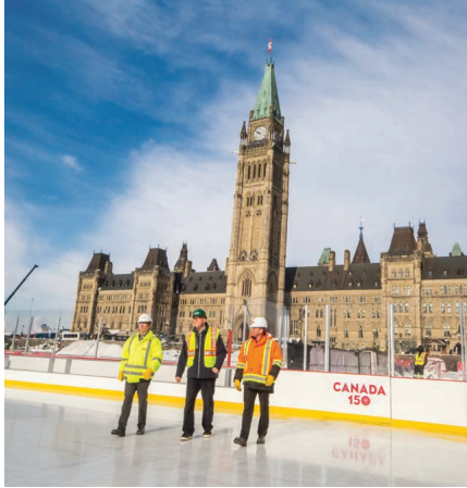
CIMCO, Battlefield and Toromont Cat teamed up to provide equipment to the Canada 150 ice rink.
