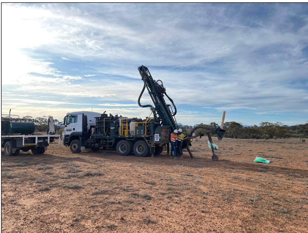
Photo. RAB drilling underway at Mt Craig
