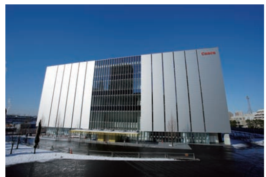
At Canon's new Kawasaki Office, CMOS sensor production and automated technology development are conducted.
