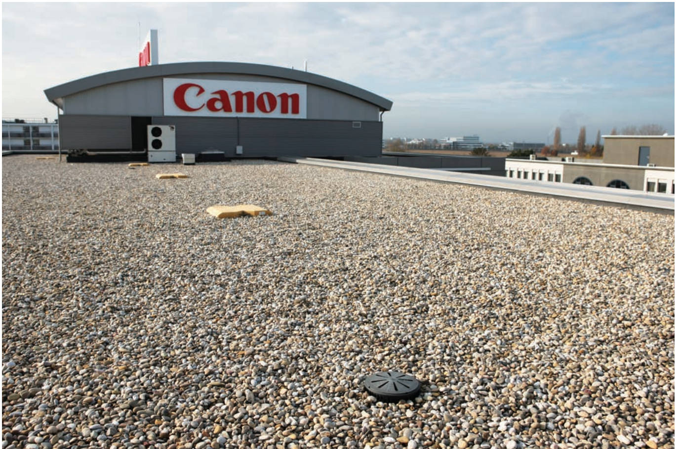
Canon strives to reduce numerous environmental burdens at its operational sites through such measures as this rooftop rainwater reuse system installed at Canon Belgium N.V./ S.A. that filters rainwater through gravel on the roof.
