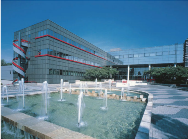
Océ's headquarters in Venlo, the Netherlands
