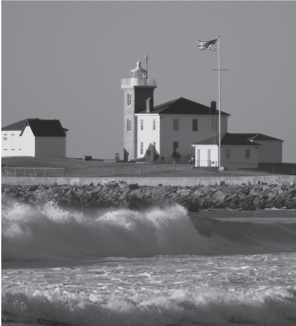
The Watch Hill Lighthouse is one of the oldest lighthouses in the United States. The original lighthouse, a 35-foot round wooden tower with ten whale oil lamps and parabolic reflectors, was built in 1807. The current granite tower was completed in 1856.
