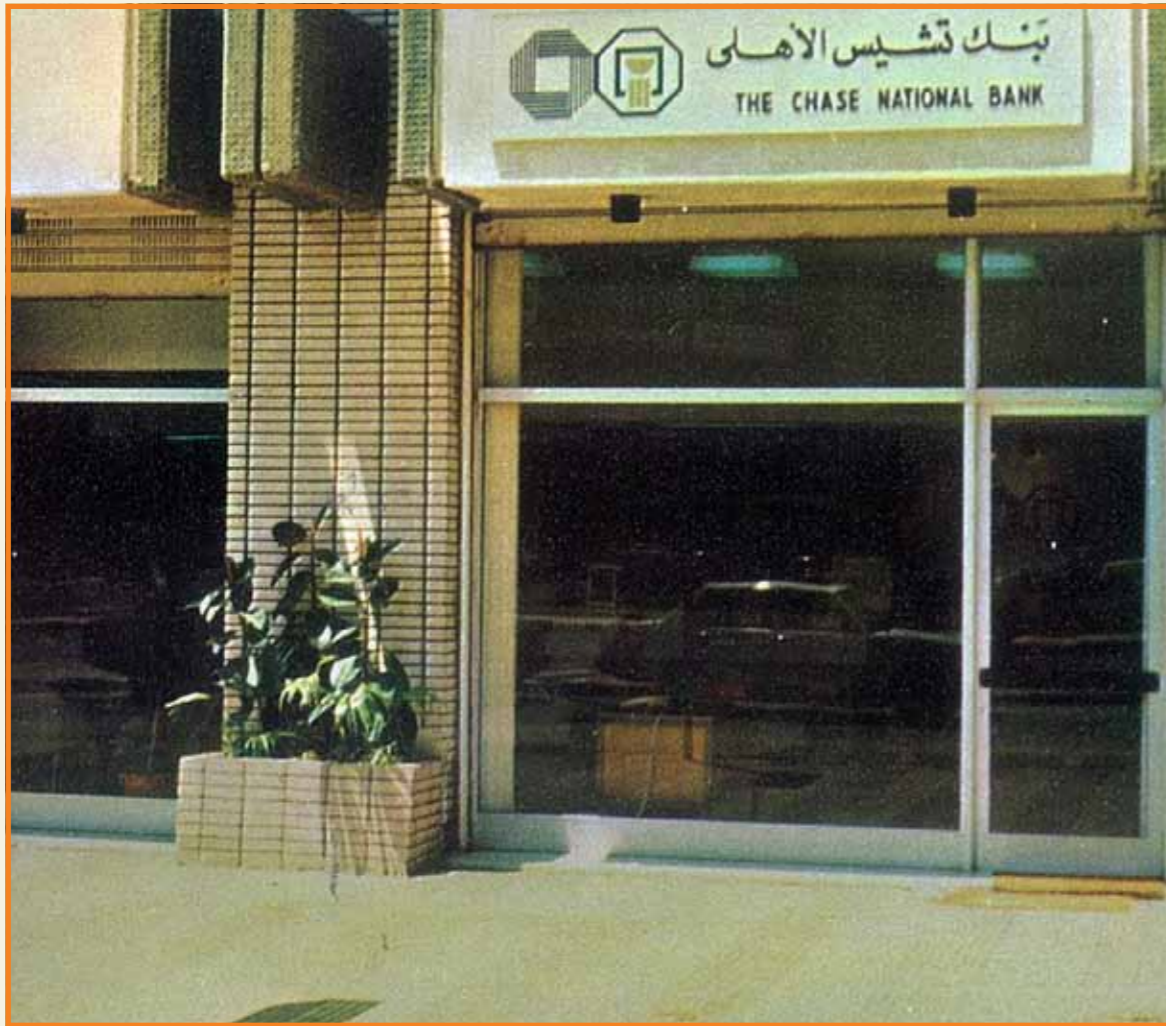
CIB owns a number of strategic subsidiaries that allow it to offer a full range of financial services, including investment banking, asset management, brokerage, research, and factoring, as well as security services.
