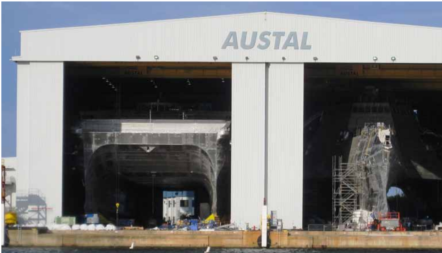
▲ The US Department of Defence's Joint High Speed Vessel and Littoral Combat Ship (LCS4) under construction at Austal's Mobile, Alabama, shipyard.
