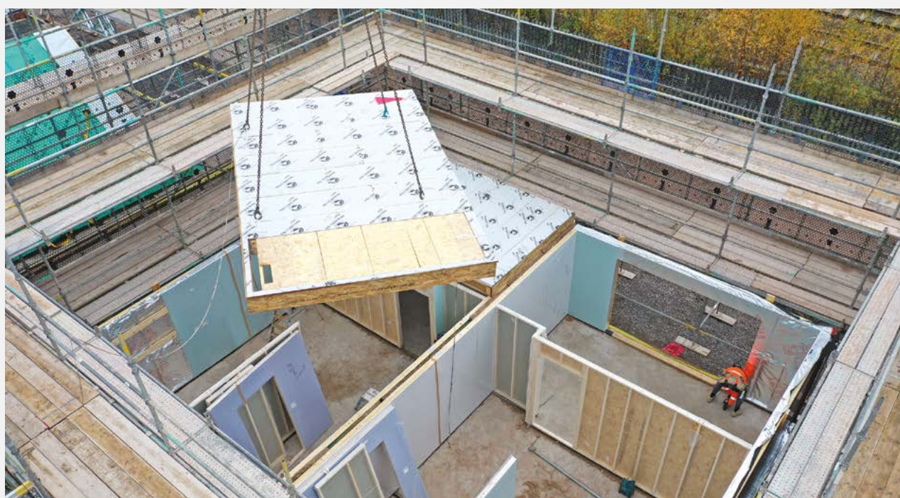
Timber frame home under construction at Beehive Mill, Bolton.
