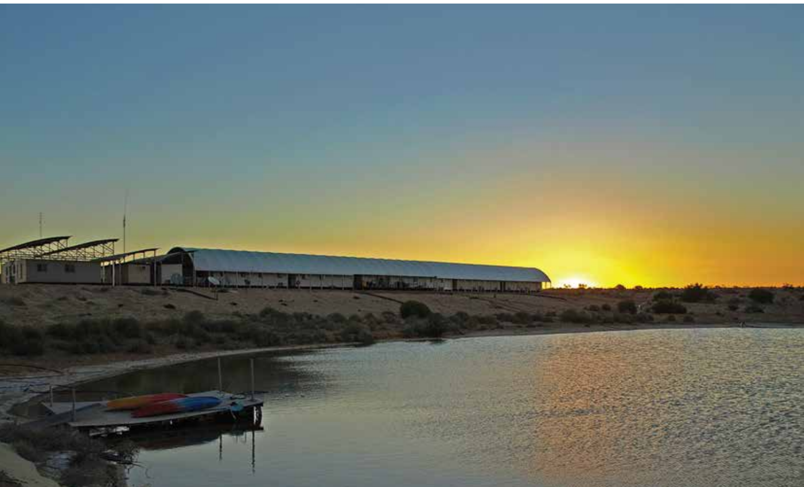
Evaporation pond and accommodation facilities, Callawonga camp, PEL 92 Cooper Basin
