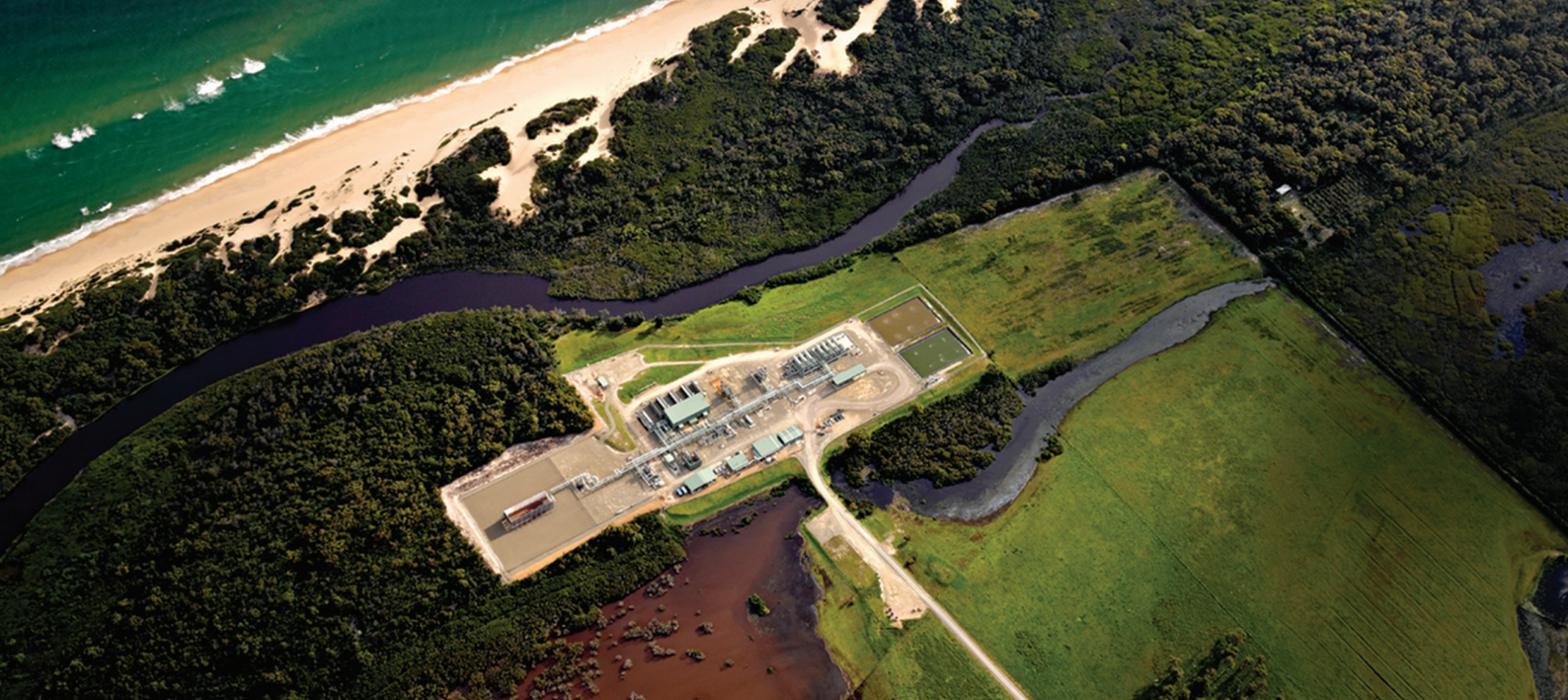
Orbost Gas Plant, Gippsland Basin, Victoria
