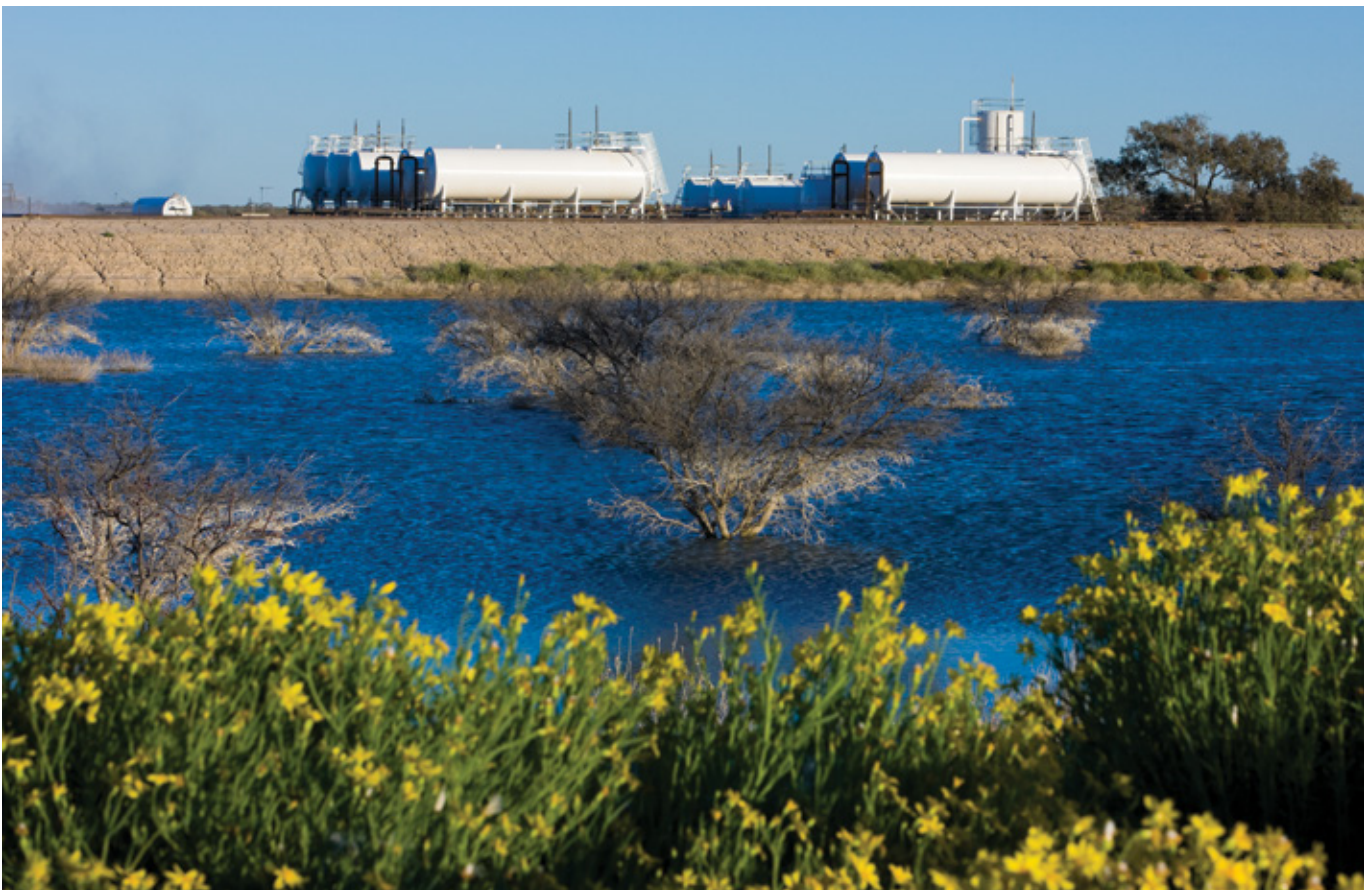
Callawonga facilities, Cooper Basin. The field was the location for six of the nine wells drilled by the company during the year, all of which were successful.
