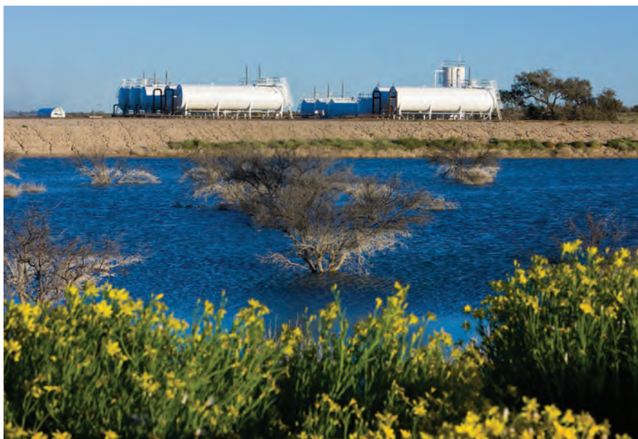
Callawonga storage facility
