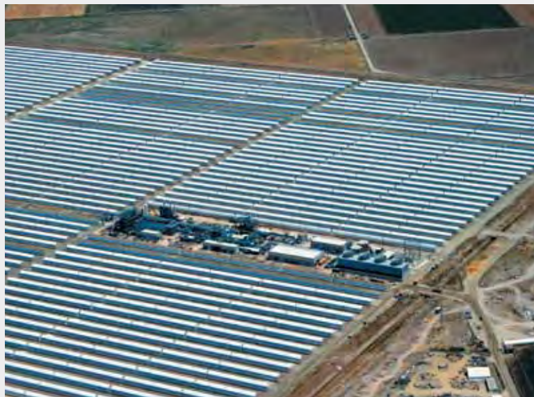
Iberese is leading the way for renewable energy production with the design of the Lebrija 1 CSP plant.
