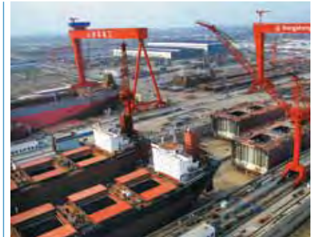
AVEVA's integrated shipbuilding solutions enable a wide range of disciplines to be addressed under one collaborative framework.
