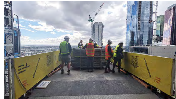
Coordinating safety in high-risk, large-scale projects - Simonds Workplace Health & Safety Team participate in a leadership workshop run by Pro-Build at Victoria University.
