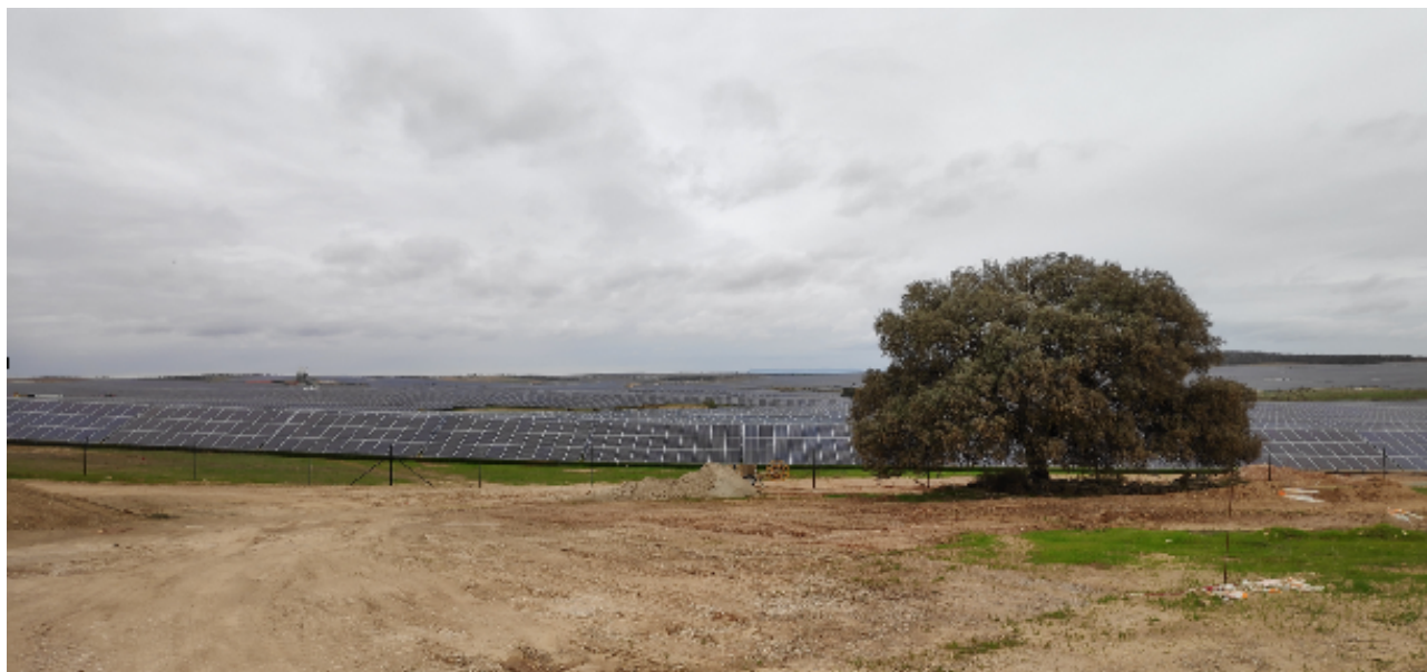
Francisco Pizarro photovoltaic power plant - Cáceres, Spain
