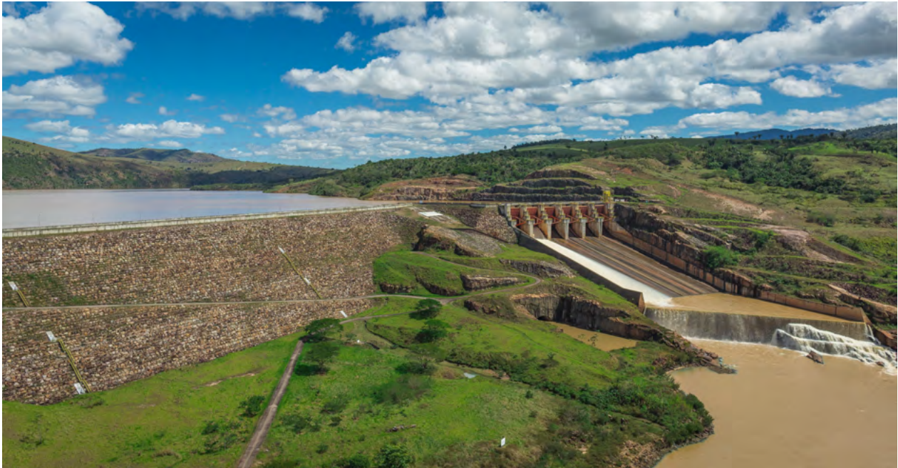
Itapebi hydroelectric plant - Bahia and Minas Gerais, Brazil
