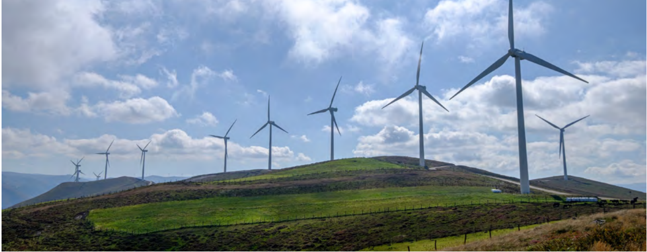
El Sedregal wind farm - Asturias, Spain
