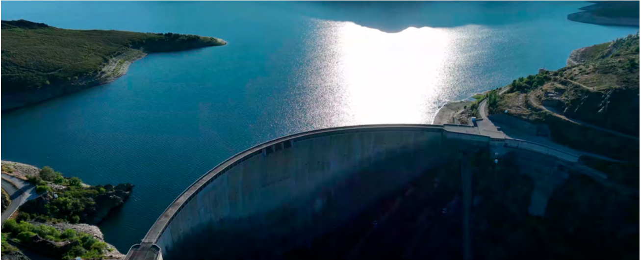
Conso hydroelectric power station, Galicia, Spain
