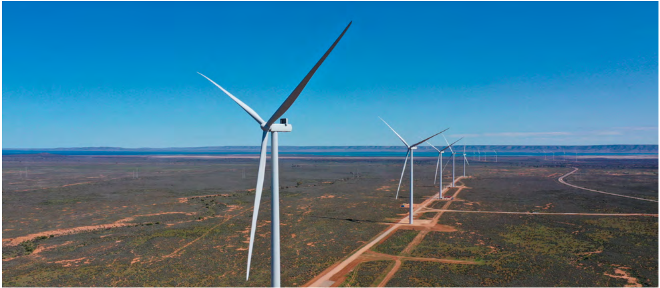
Port Augusta wind farm, Australia
