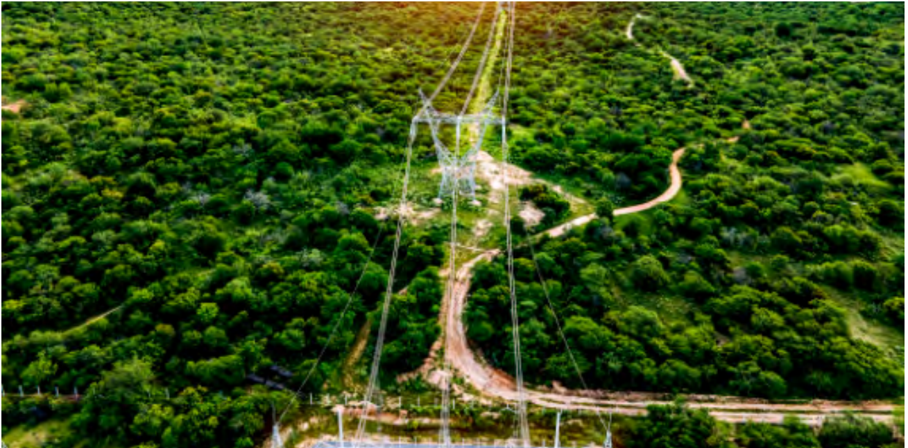
Santa Luzia transmission Line, Brazil
