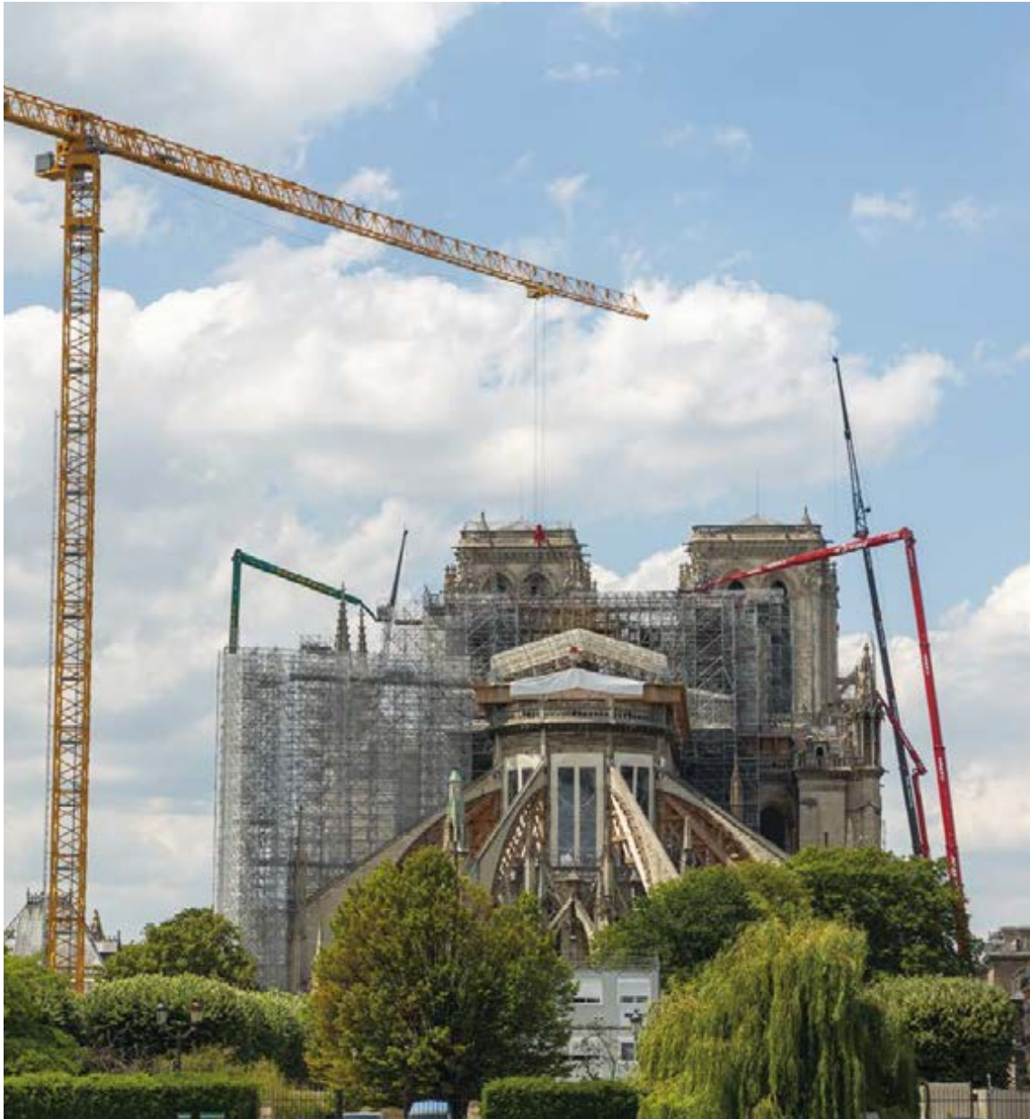
Restoration of Notre-Dame de Paris Cathedral. Site safety and consolidation phase.
