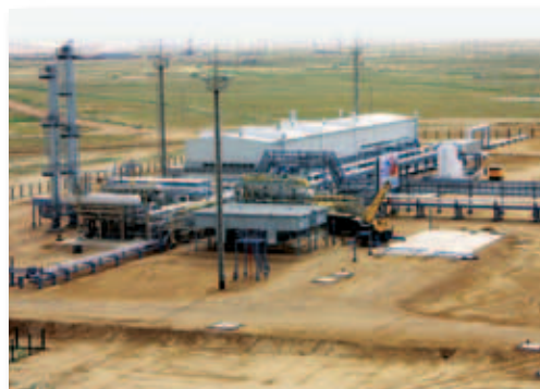
Gas processing facility built for a customer in Kazakhstan
