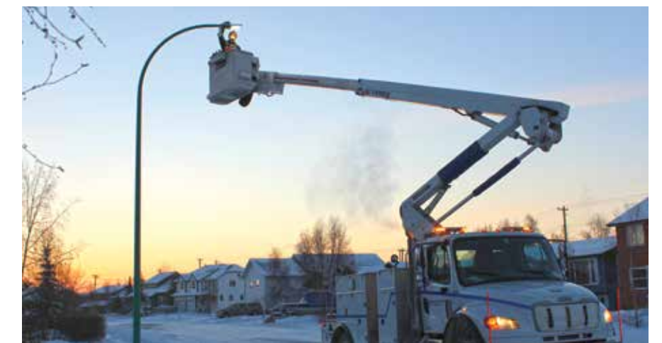
A Northland Utilities Powerline Technician inspects a recently installed LED streetlight in Yellowknife, NWT.
