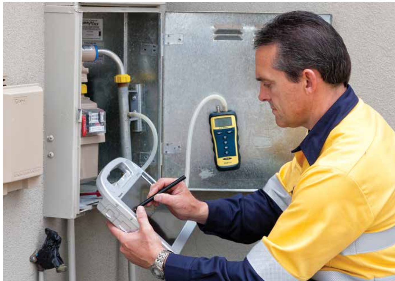
Pat During, Gas Distribution Officer, ATCO Gas Australia, is conducting a meter read using the Field Mobility System developed in conjunction with ATCO I-Tek Australia.
