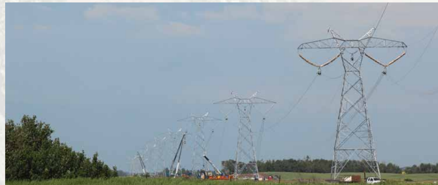
The Eastern Alberta Transmission Line stretches along the east side of Alberta and comprises 485 km of 500 kilovolt, direct current line and associated converter stations and facilities. The project will reinforce the reliability, increase the capacity and improve the efficiency of Alberta's electricity grid.
