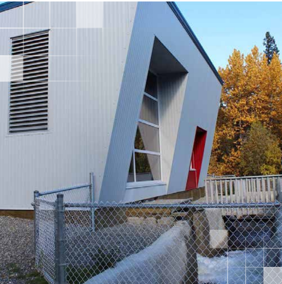
Fish Lake Hydro One is the Yukon's first hydro power facility, dating back 64 years. In 2014, ATCO Electric Yukon completed the redevelopment of the station.
