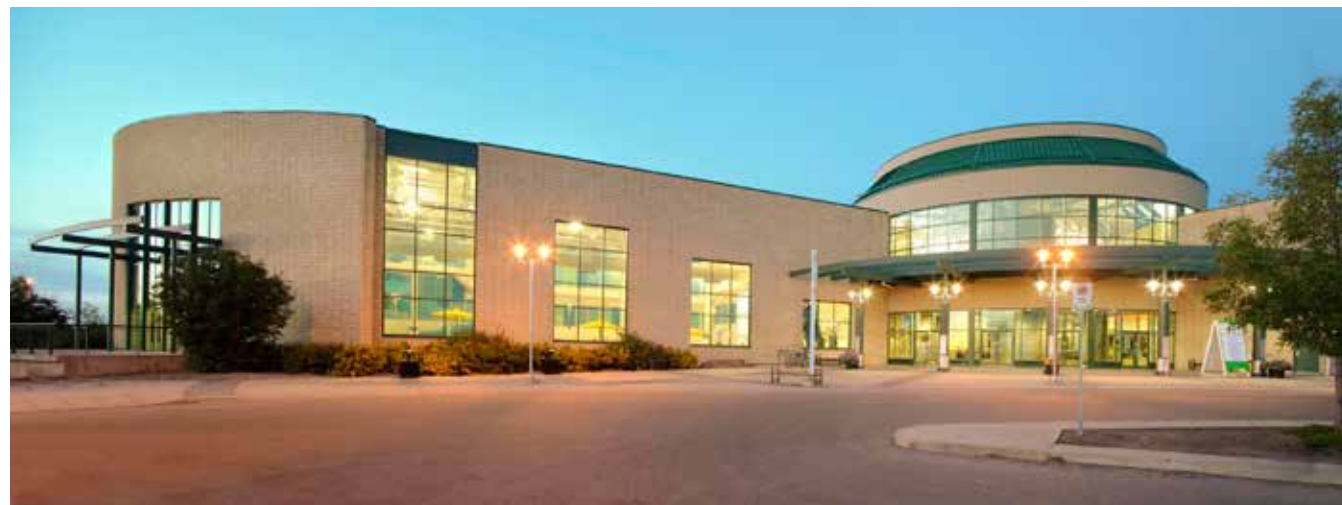
The Collicutt Centre, a 260,125 sq. ft. recreation facility in Red Deer, Alberta, was one of the first customers to sign up for ATCO Gas's Combined Heat and Power program. The program incorporates technology that increases energy efficiency and reduces energy costs and greenhouse gas emissions.
