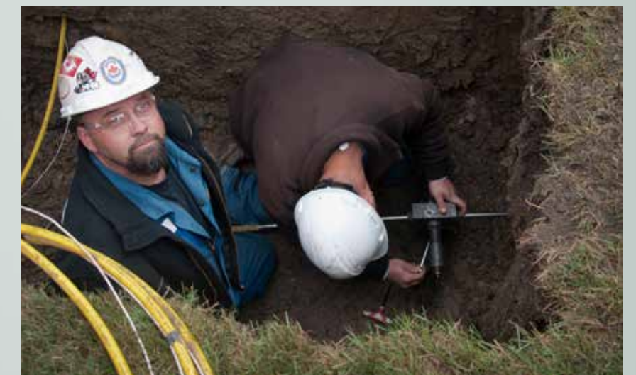
Through the IdeaWorks 2.0 program, ATCO Gas employee Paul Kendall, left, submitted an idea for a new tubing tool that is now being rolled out to employees and contractors throughout Alberta. The tool provides a safe way to connect two gas lines while gas is still flowing.
