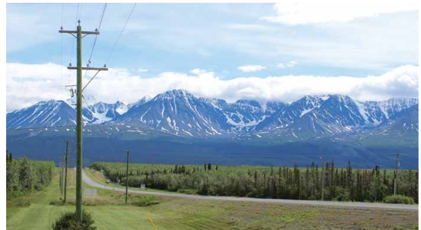
A section of distribution line outside of Haines Junction, overlooking St. Elias Mountain in the Yukon. ATCO serves more than 17,000 customers in the territory.
