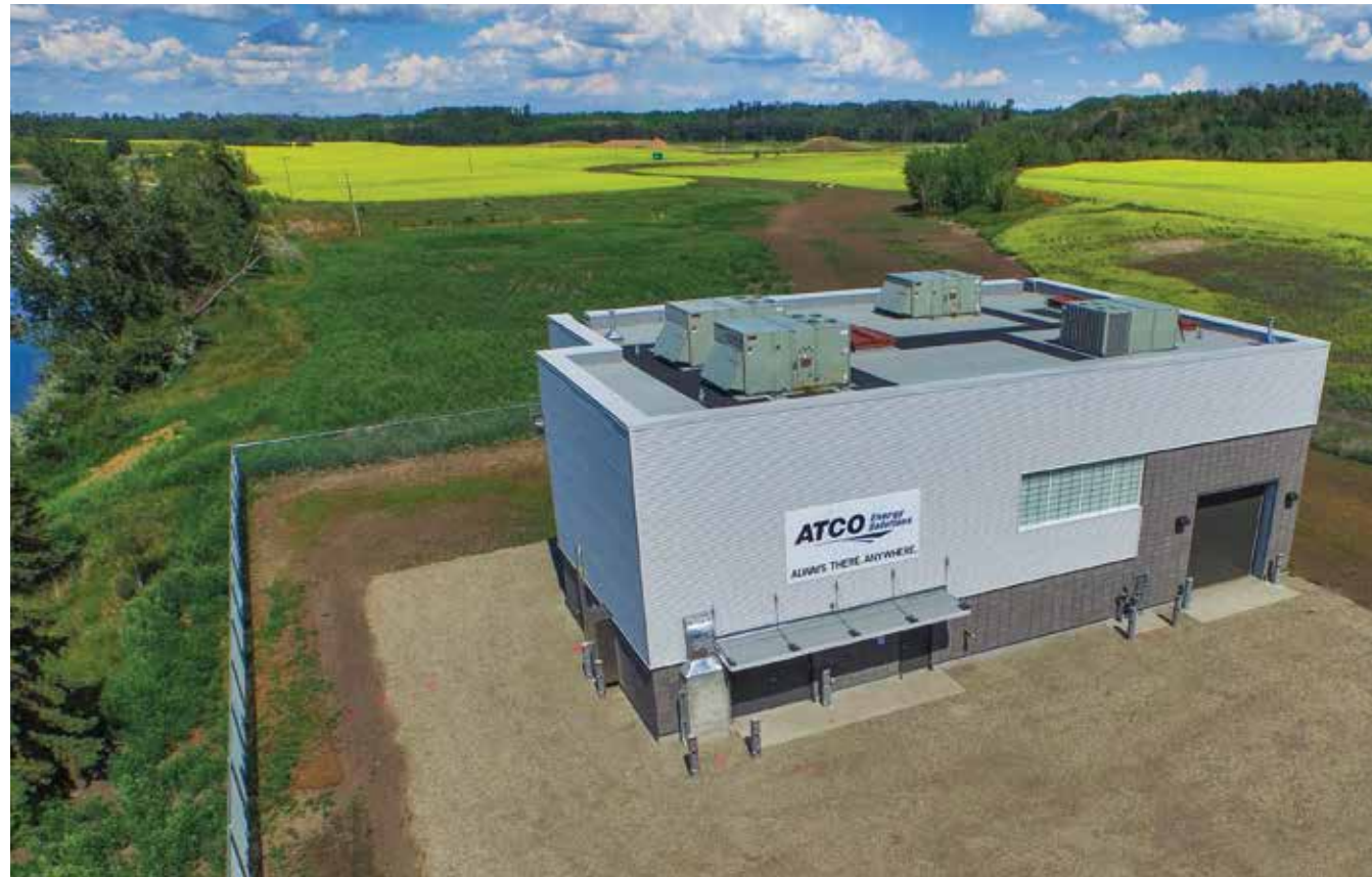
ATCO Energy Solutions' new industrial water pump station, strategically located on the North Saskatchewan river in Alberta's Industrial Heartland.
