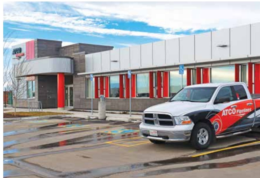
In December 2015, ATCO Pipelines opened its new 19,000 sq. ft. South Operations Centre in Airdrie. It features 12,000 sq. ft. of office space, room for material and equipment storage, and two drive-through vehicle bays and a storage bay.
