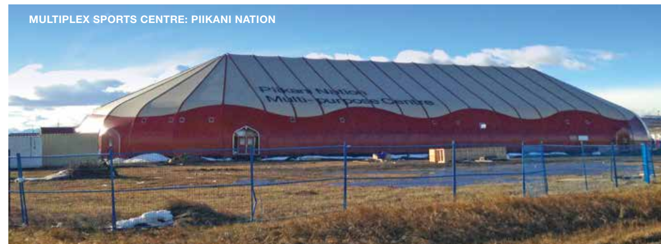
When complete, the Piikani Nation's state-of-the-art 36,000 sq. ft. multiplex sports centre will be the largest project in ATCO Sustainable Communities' history.
