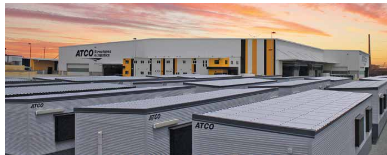
ATCO was awarded a further contract to design, manufacture and install an additional 435 modular units with Bechtel on the Chevron-operated Wheatstone Project in Western Australia. The units were manufactured at ATCO's Kwinana Manufacturing facility (above).
