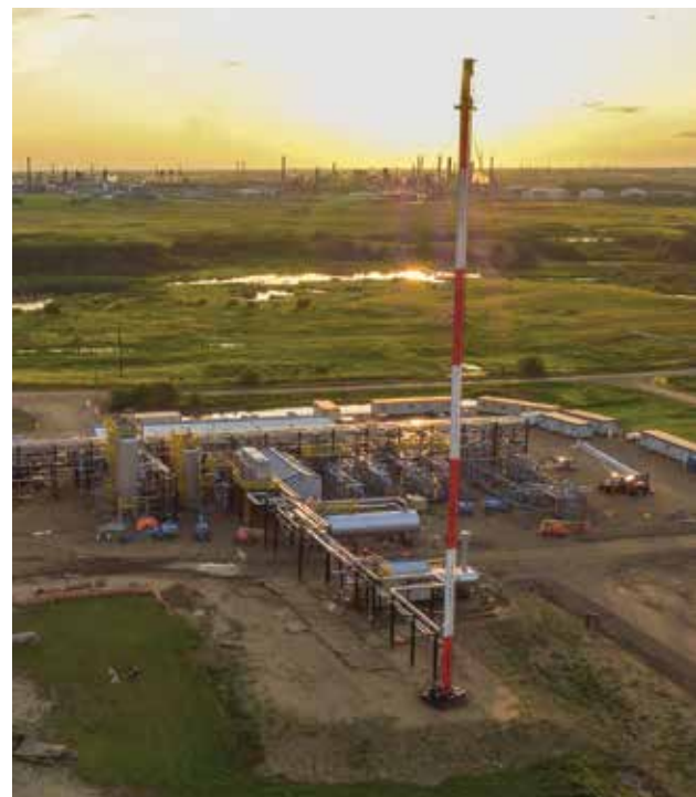
Our salt cavern facility at the ATCO Heartland Energy Centre allows us to leverage our industrial water infrastructure in the area to wash two caverns simultaneously which shortens development time. The central location also provides our customers with transportation options to solve the logistical challenges of moving product to market or securing it to avoid processing interruptions.
