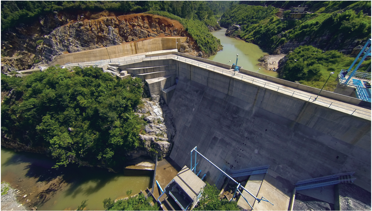
Electricidad del Golfo Hydroelectric Power Station
