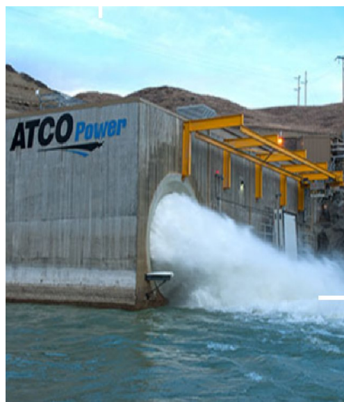
Oldman River Hydroelectric Plant
