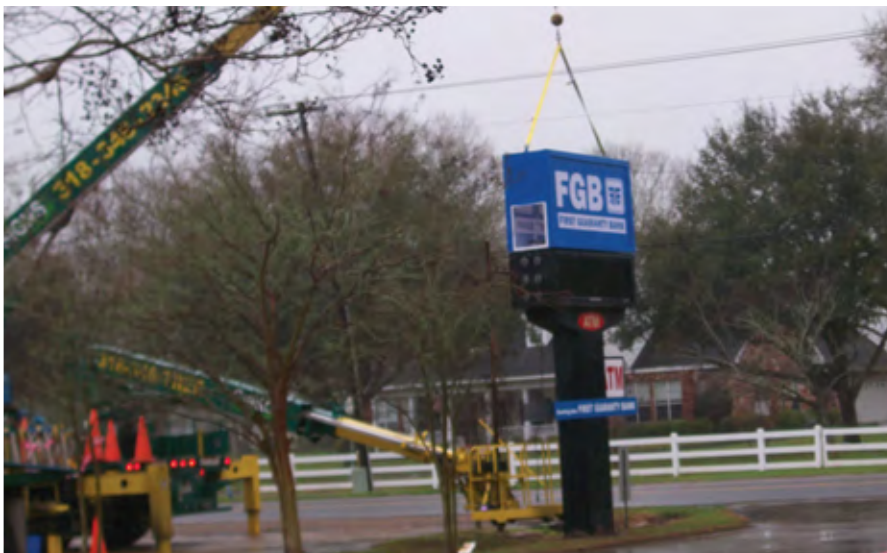
First Guaranty Bank signage being installed at Hessmer, LA branch.
