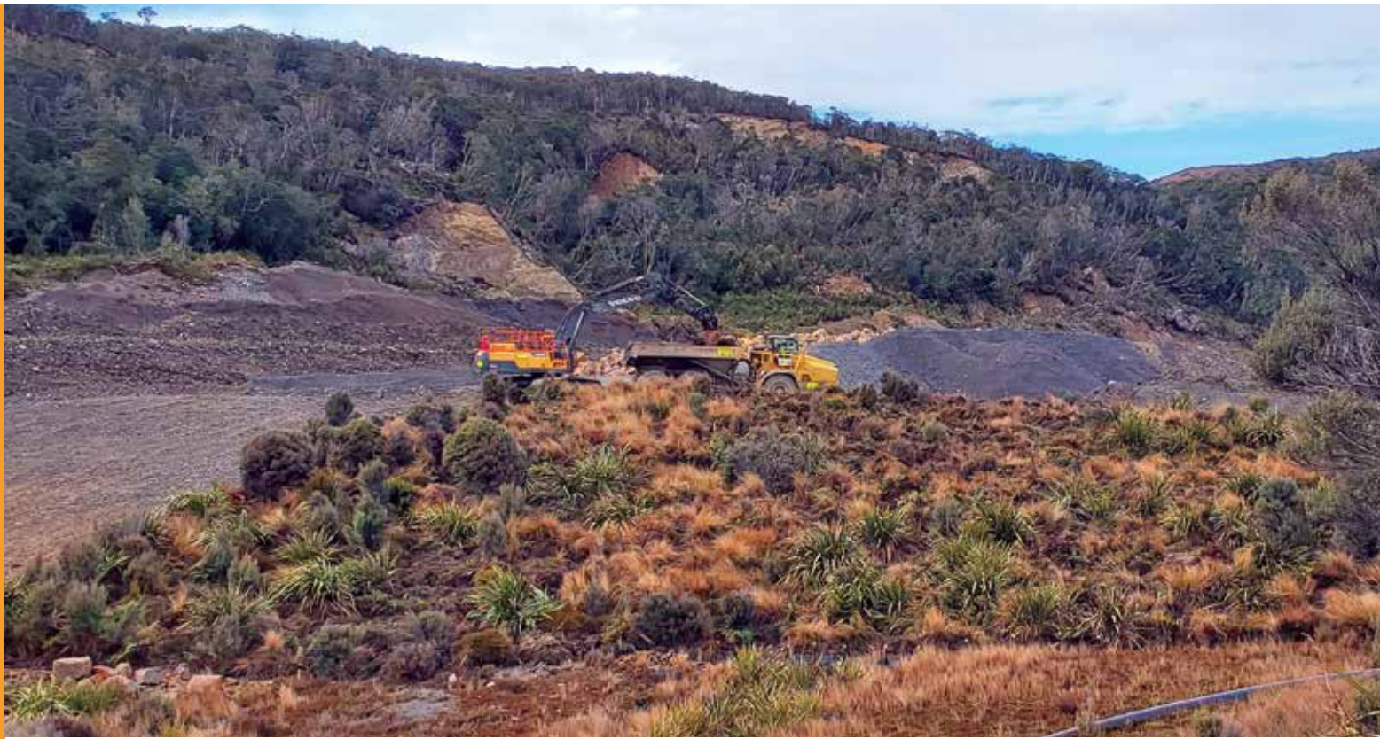
Red tussock being relocated back to Cypress mine by vegetation direct transfer
