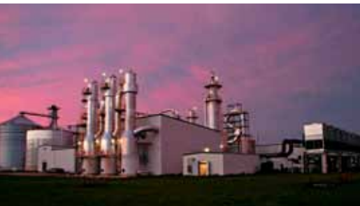
Green Plains ethanol facility in Superior, Iowa
