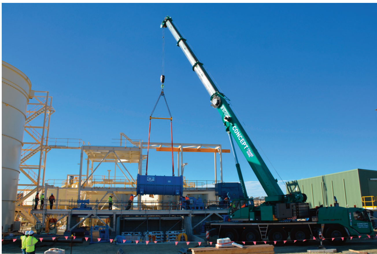
Figure 7: IsaMill™ craned into position 15 August
