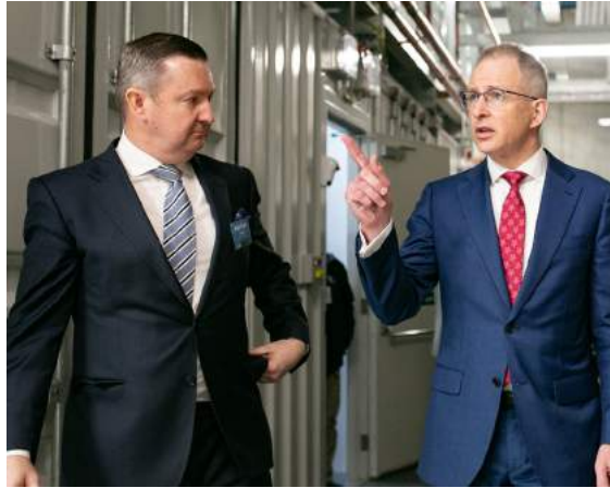
The Hon Paul Fletcher, Minister for Communications, Cyber Security and the Arts and Mr Madden at the opening of DXN-SYD01
