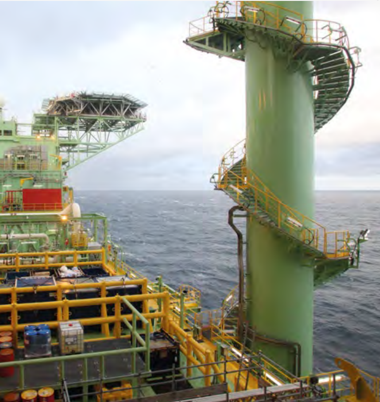
Left: The BW Catcher FPSO
