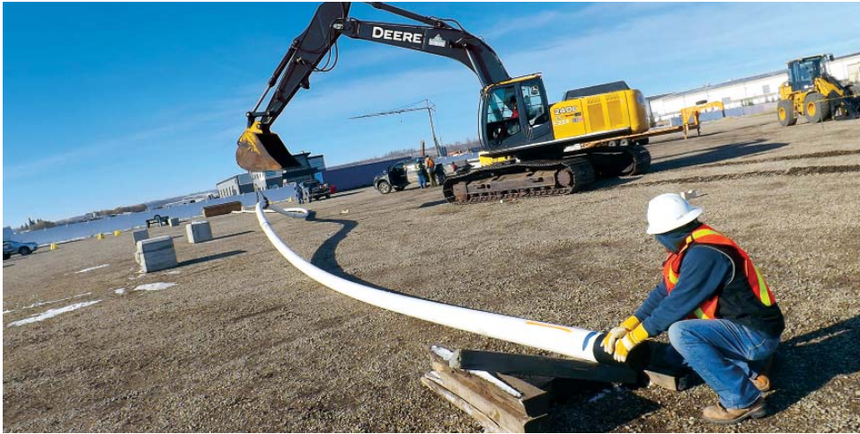
Left: FlexPipe entered the large diameter composite market space with the first field trials of FlexFlow™ 6-inch discreet length composite line pipe.
