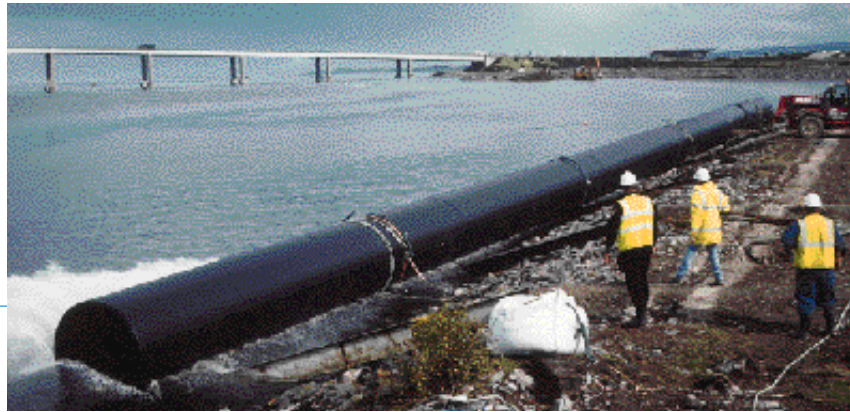
Asset Weholite HDPE pipe chosen for 650 m long sea outfall in Scotland.
