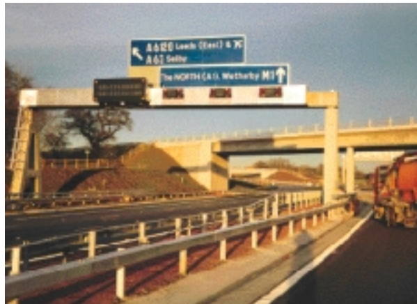
Sign gantry and bridge parapet supplied by Varley & Gulliver and motorway barrier supplied by Hill & Smith on the new A1/M1 link in Yorkshire
