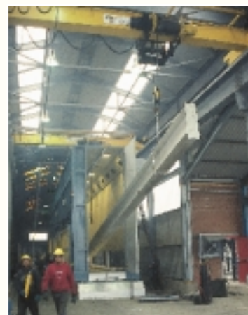
Structural beam being dipped at the 18 metre modern galvanising facility at Joseph Ash.
