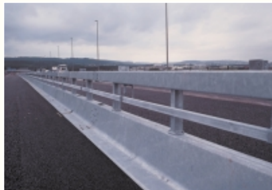
Varioguard — in permanent position on the Avonmouth Bridge.
