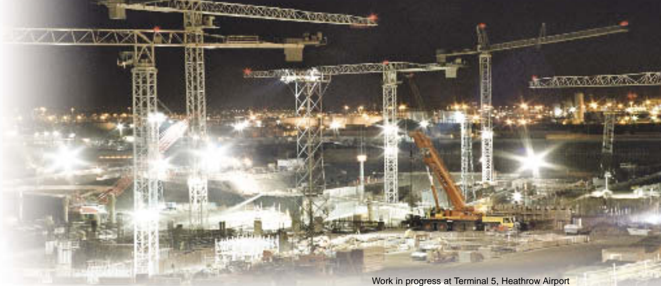
Work in progress at Terminal 5, Heathrow Airport
