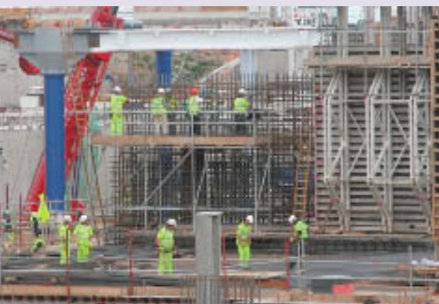
Reinforcing bar supplied to Express Reinforcements' joint venture at Terminal 5, Heathrow.
