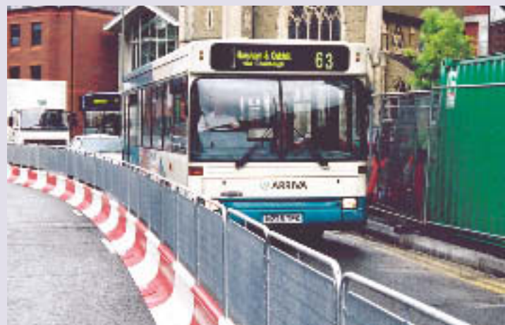
The “Mass” pedestrian and vehicle safety system, in use at Guildford Town Centre.
