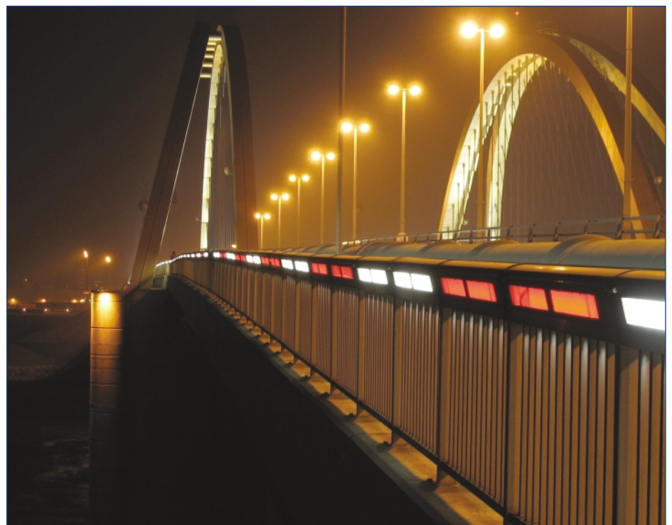
Right: Varley & Gulliver's aluminium parapets on the Shaikh Khalifa Bridge, Bahrain.
