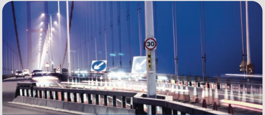
Asset Varioguard emergency crossing points on Humber Bridge.
