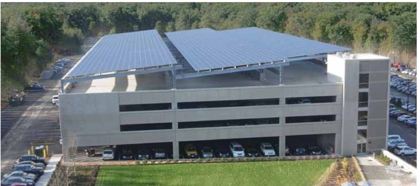
Staples garage at Framingham Massachusetts where our US galvanizer Voigt & Schweitzer galvanized the steel framework comprising 272 tonnes.
