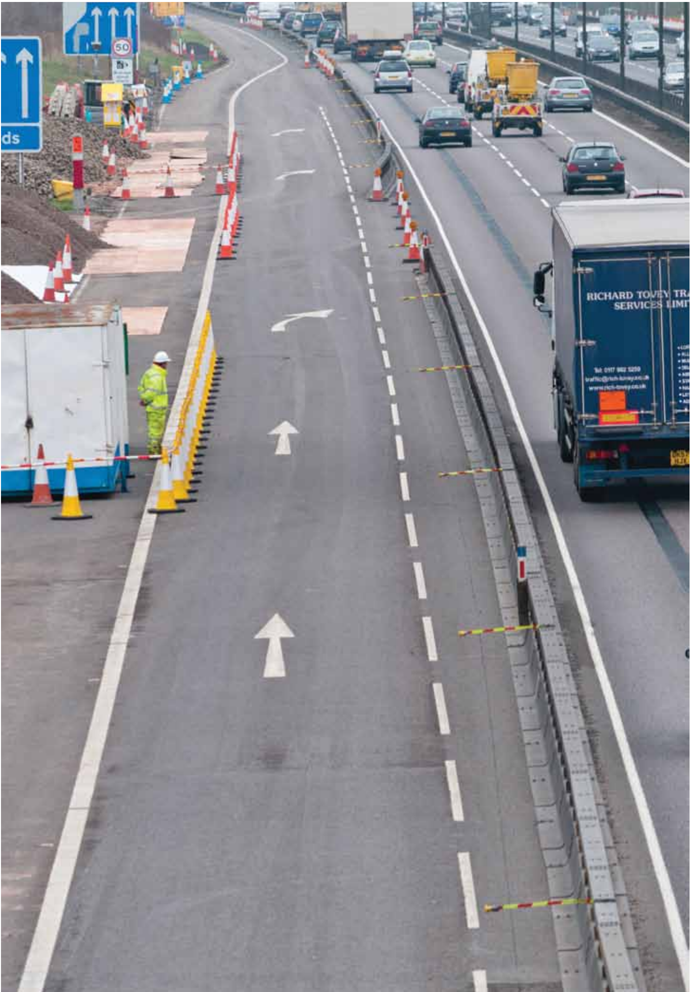
Deployment of our Varioguard barrier system on the M4/M5 Almondsbury interchange, Bristol for a managed motorway project undertaken in the summer of 2012.
