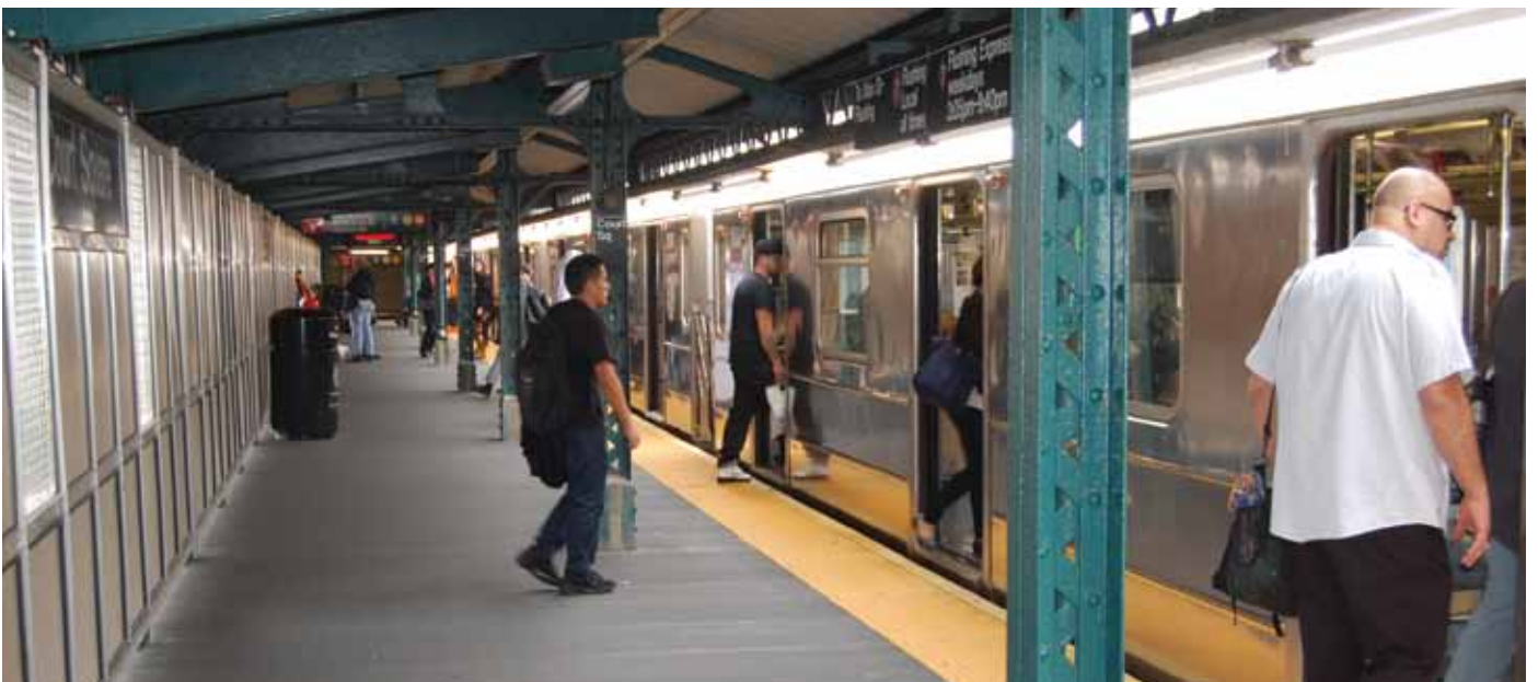
'GRP' SUPERDECK mass transit decking installed at 45th Road, Courthouse Square rail station, New York, which replaced the existing concrete platform with a lightweight limited maintenance decking system. The platform comprised 13,000 square feet of SUPERDECK which was manufactured and supplied by our US company Creative Pultrusions Inc.
