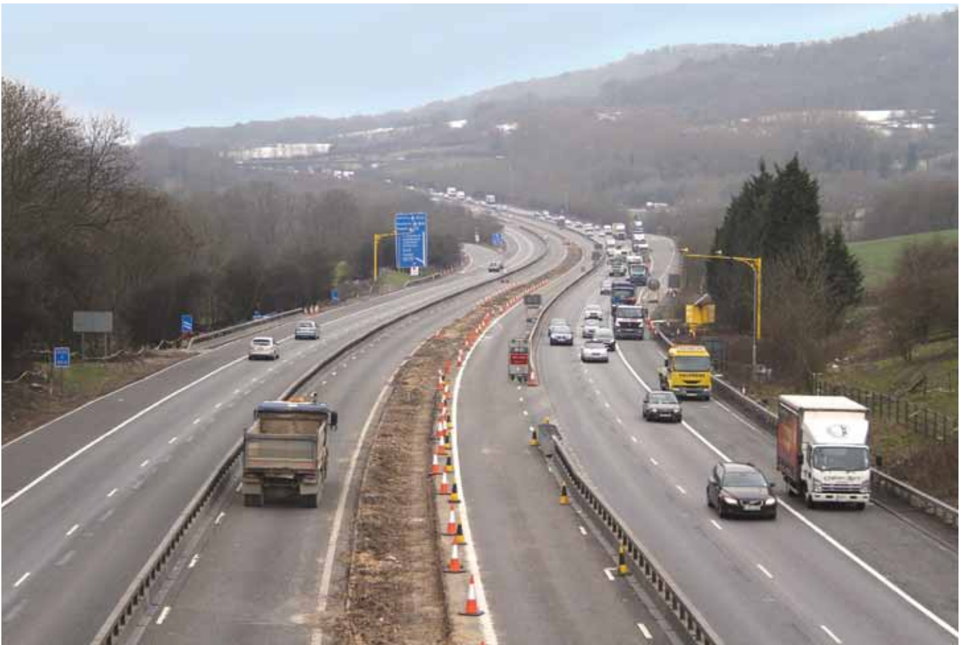
Varioguard in use at junctions 5 to 7 of the M25 for the central reservation work of the managed motorways contract.
