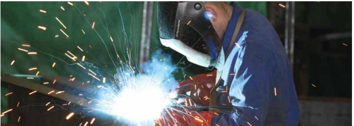
Welding of industrial flooring at our Lionweld Kennedy Flooring business, Middlesbrough.
