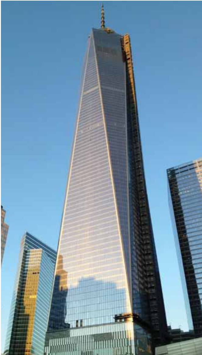
Bergen pipe supports used in the Freedom Tower, New York City and steel structure to the outer area of the upper floors galvanized by V&S Galvanizing.
