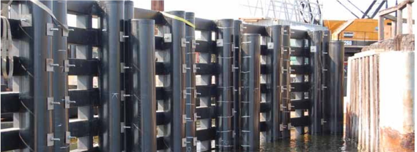
Creative Pultrusions fender piling for the New Jersey Water Authority.
