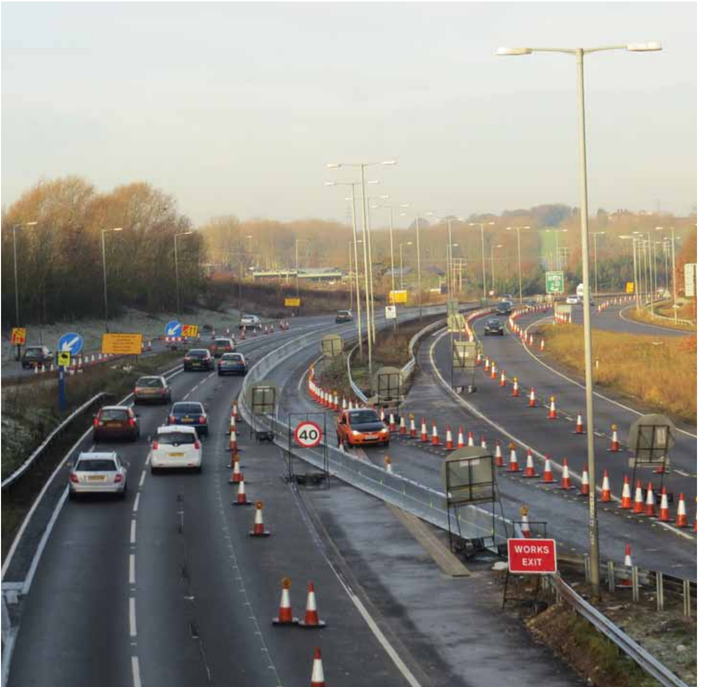
Zoneguard temporary road barrier on the A14 Kettering Bypass.
