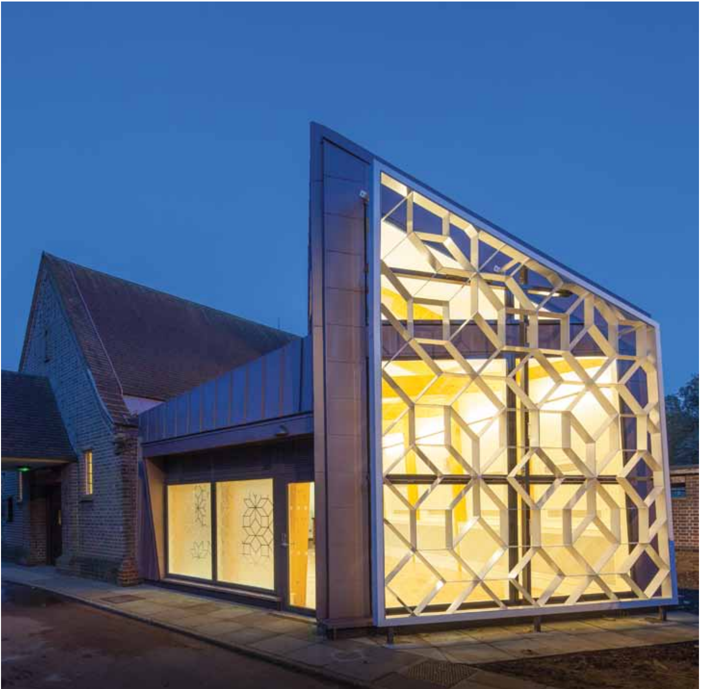
Medway Crematorium showing the ornate galvanized window structure.
