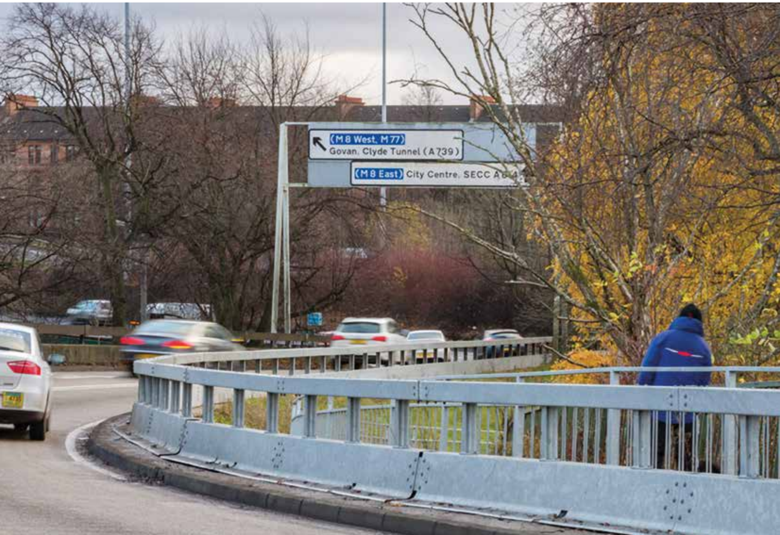
Top: ZoneGuard installed on E4 at Häggvik north of Stockholm, at the start of the new Stockholm ring road. Below: Single-sided Varioguard installed on the Clydesdale Expressway, Glasgow.
