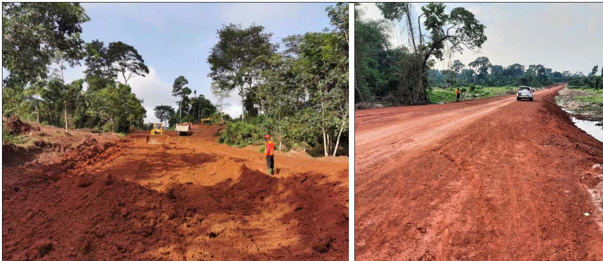
Figure 10: Abujar site access road in construction
