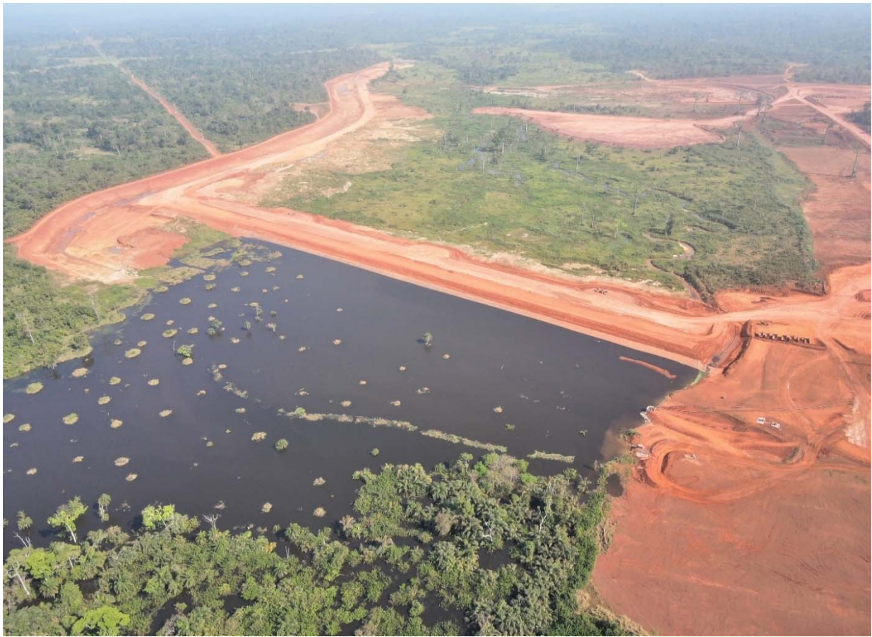
Figure 7: Water storage dam and diversion channel
