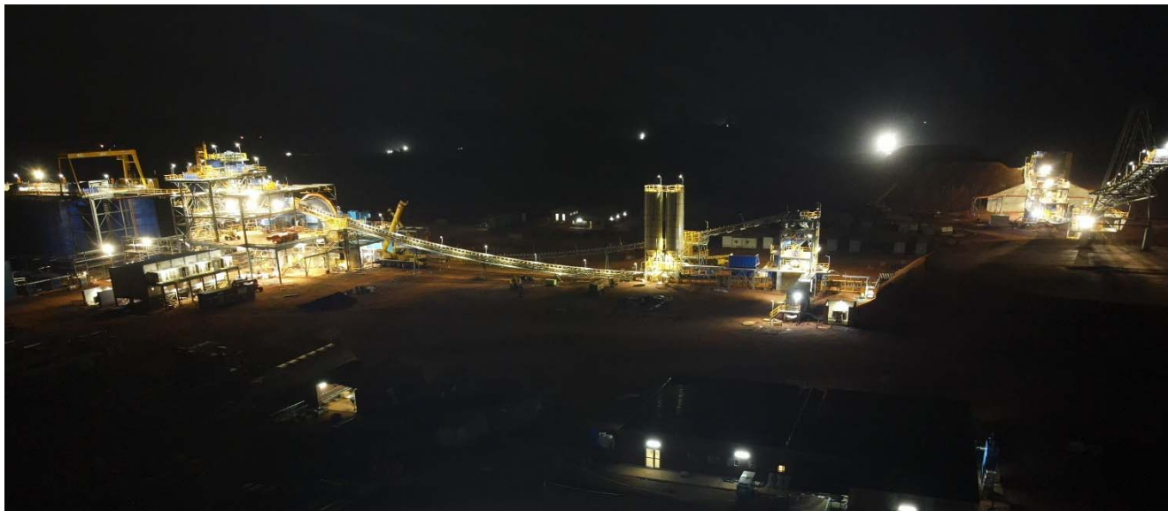
Figure 2: Abujar Plant at night
