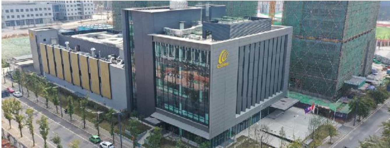
Our new manufacturing facility in Chengdu, China.
