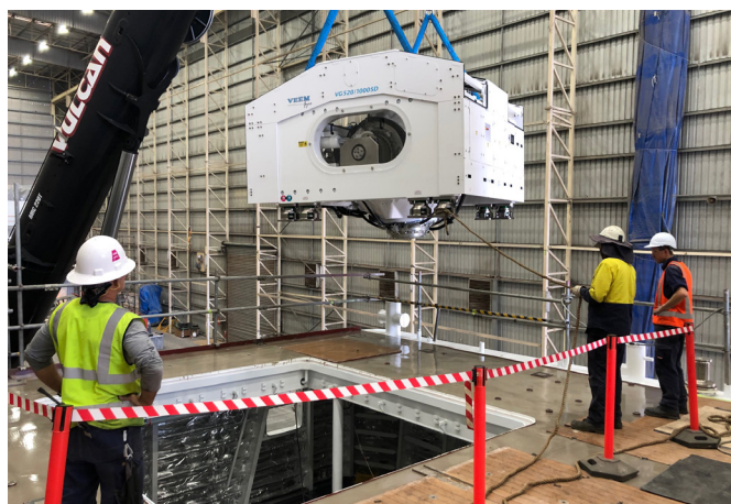
Figure 5: A VEEM Marine VG520SD being installed into MV Umbra
