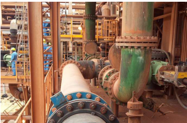
Figure 3: VEEM forever Pipe in-situ (green).
