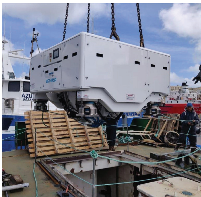
Figure 7: A VEEM Marine VG140SD being lowered into Fish and Fish Ltd. workboat M/V Emmaya.
