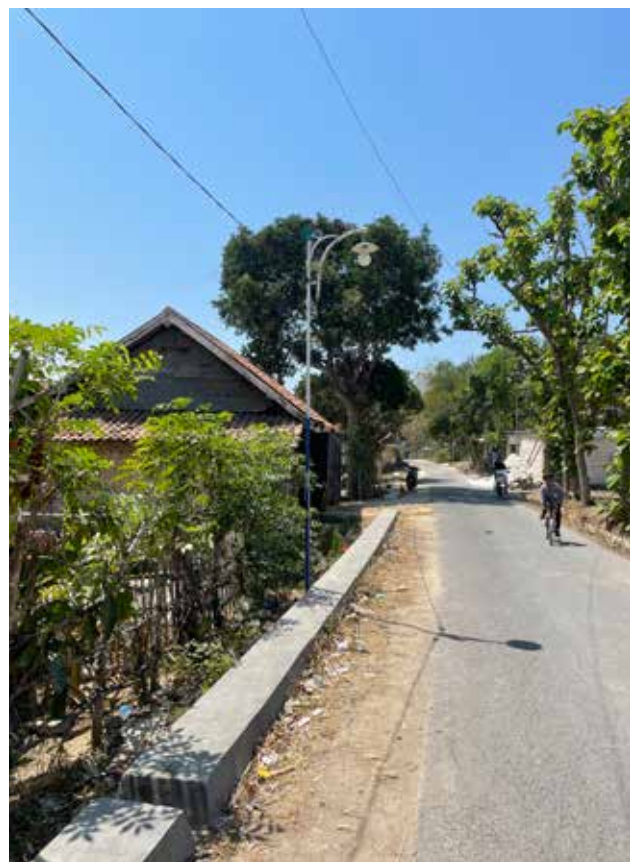
Sampang PSC: village external lighting installation
