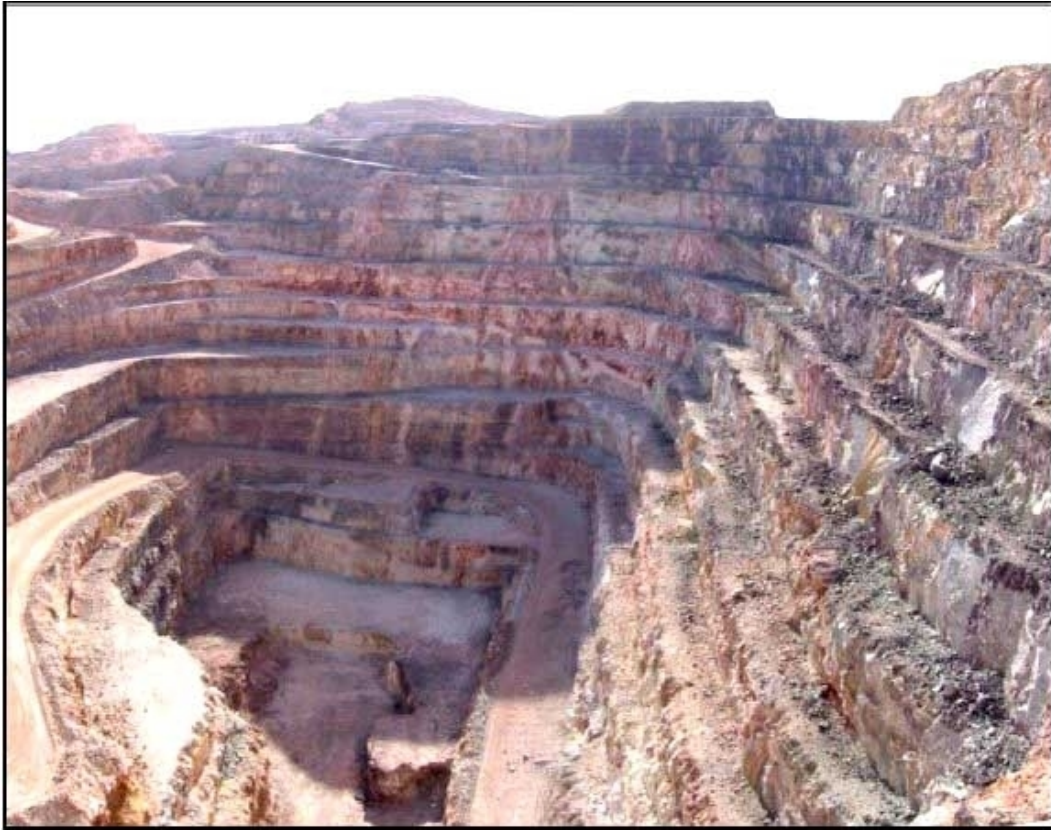
The photograph above shows the east view of the Dumbo open pit showing the deepest of the past workings. The photograph below shows the leach pads, north of the Dumbo pit.
