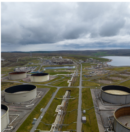
View of Central Avenue Sullom Voe Terminal
